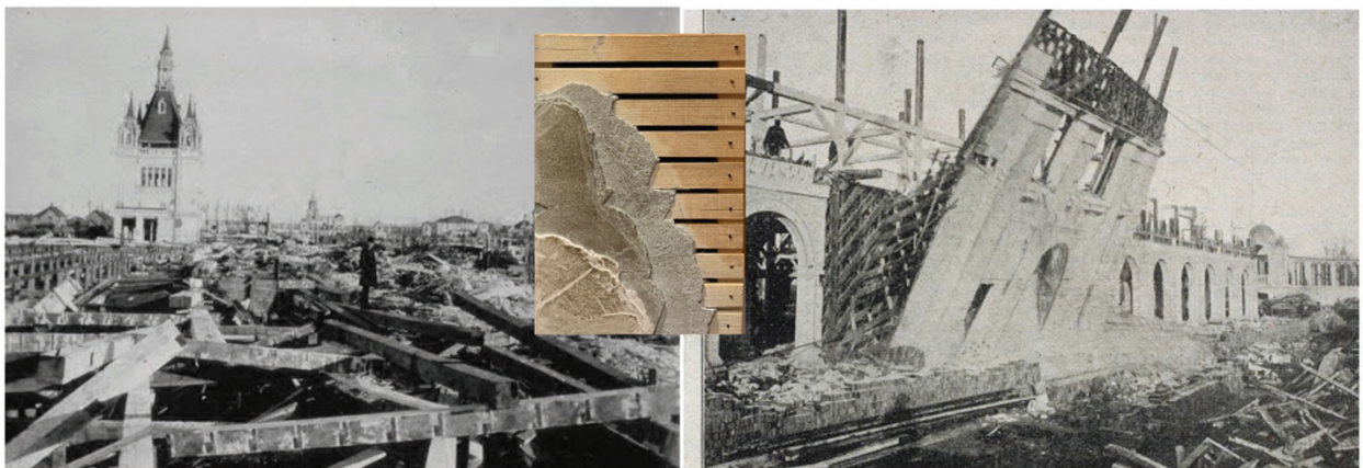
Left & Right: Pictures of the exposition's demolition. Images courtesy of trans-mississippi.unl.edu and northomahahistory.com . Center: Image of laths and staff construction used for building façades. Picture taken by the author at the Durham Museum, Omaha, NE.
